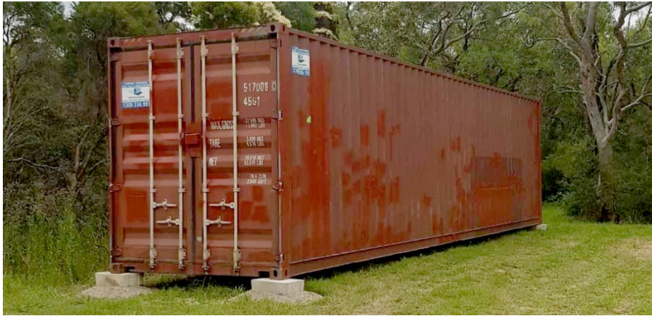
Containers lifted from the ground on blocks
